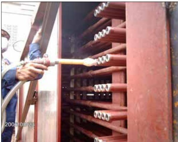
**VpCI®-309 Nitrite Free Powder** is a Vapor phase Corrosion Inhibitor powder for corrosion protection of ferrous metals in recessed areas, interior cavities, and voids. VpCI®-309 provides an extremely efficient dry method to protect metals within an enclosed space. The VpCI® vaporizes and adsorbs on all metal surfaces reaching all exposed areas including recessed sections and interior cavities. VpCI®-309 SF, a silica-free version, is available upon request.
